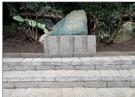
After – the newly restored memorial.
