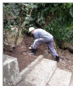
Shawfong excavating the garden.
